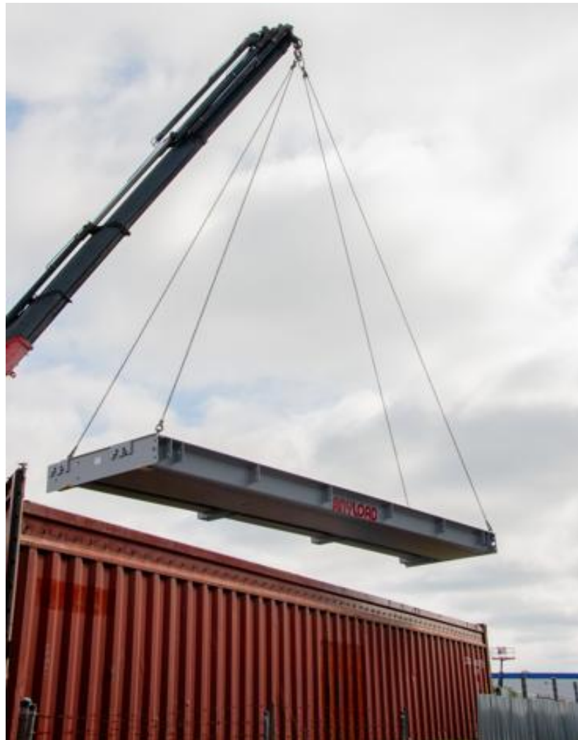
Figure 6 - Method A: Lifting each scale body with provided eyebolts.
